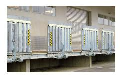
All models are available in either stationary or sliding versions. A maintenance-free spring system allows operation by one single person even on the higher load capacity models. An automatic lock retains the lip in a safe parked position when not in use, preventing any unintentional movement of the loading lip.
